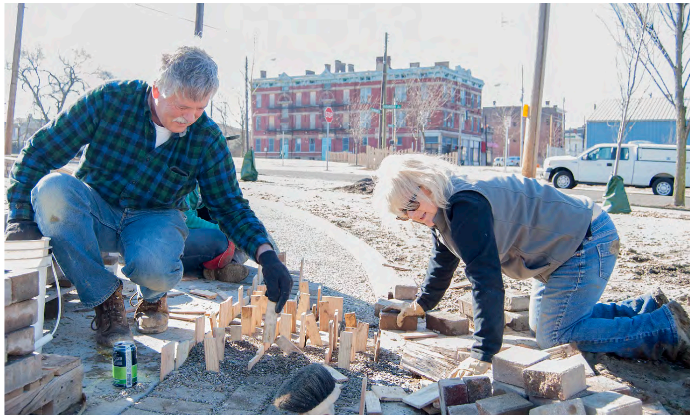
Community supporters, Chris and Sheila DeSimio , laying pavers for the pervious sidewalk.
