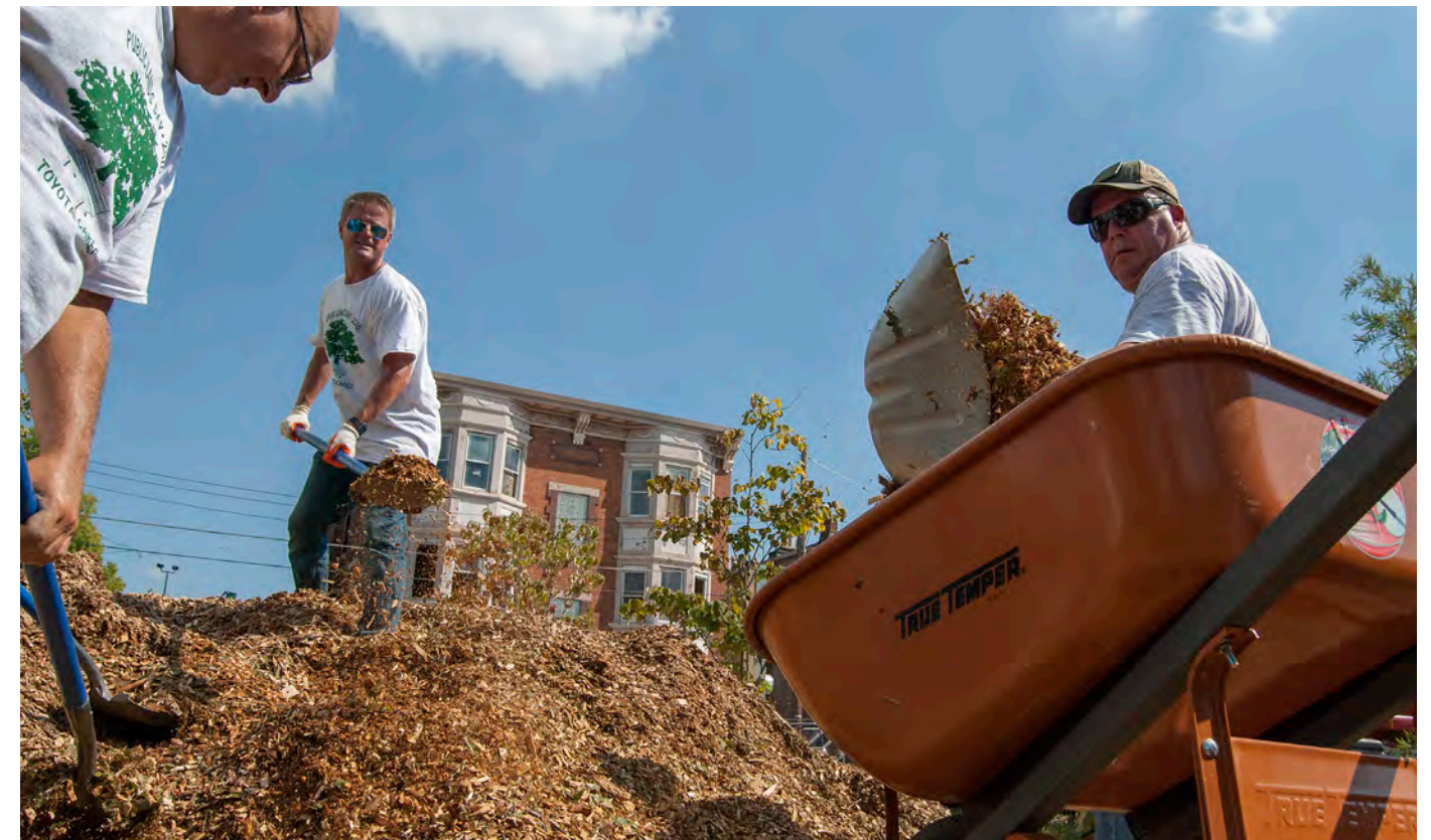
The hard-working crew from Toyota | Cincinnati Region building the dog-walking trail.
